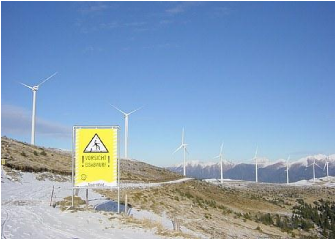
Figure 28. Warning against shedding ice fragments at Tauernwindpark in Austria. Photo from http://www.tauernwind.com .
