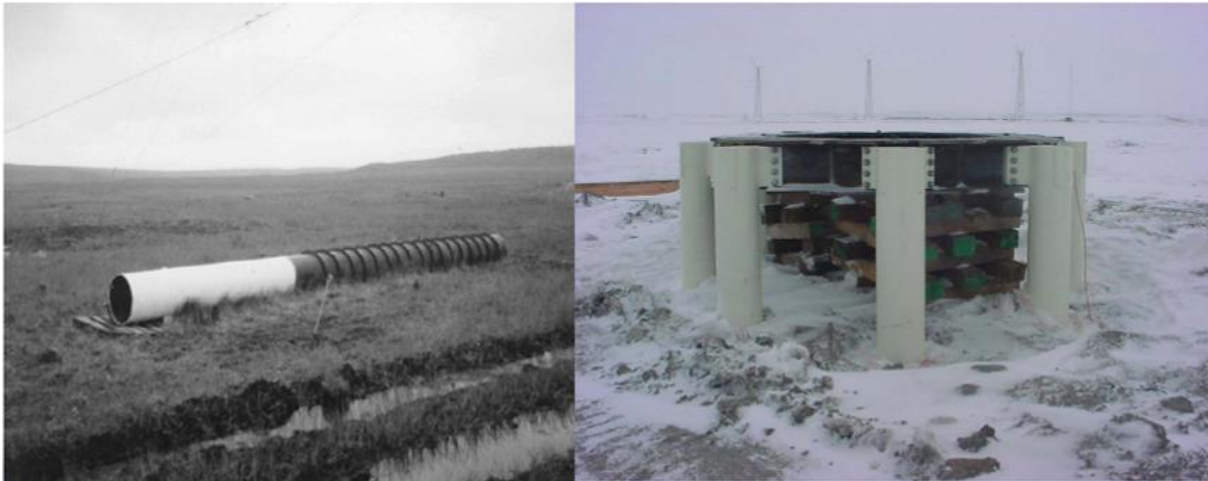
Figure 5-2: Freeze-back pylons used for turbine (and other) foundations in permafrost areas. Photo credit, Northern Power Systems, USA
